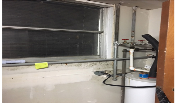
Mold at Gyp board
