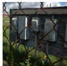
Closeup of Disconnects
