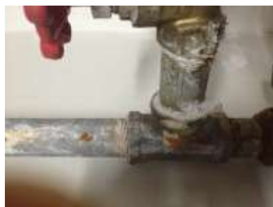
Corrosion at valves and fittings
