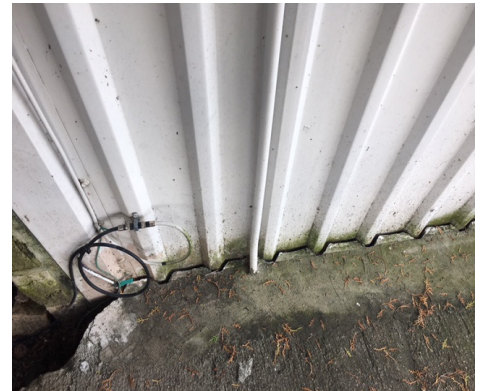
Sidewalk poured against north wall
