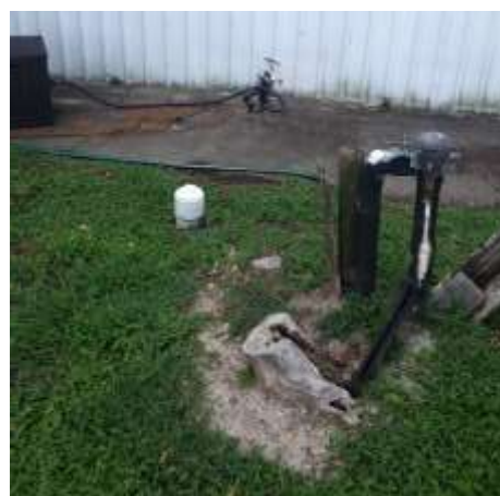
Exterior Hose Bibb, Sanitary Clean Out, Landscape Backflow Preventer
