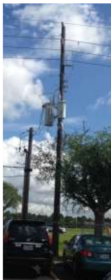
Pole Mount Transformer
