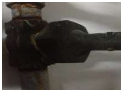
Main Water Shut off Valve
